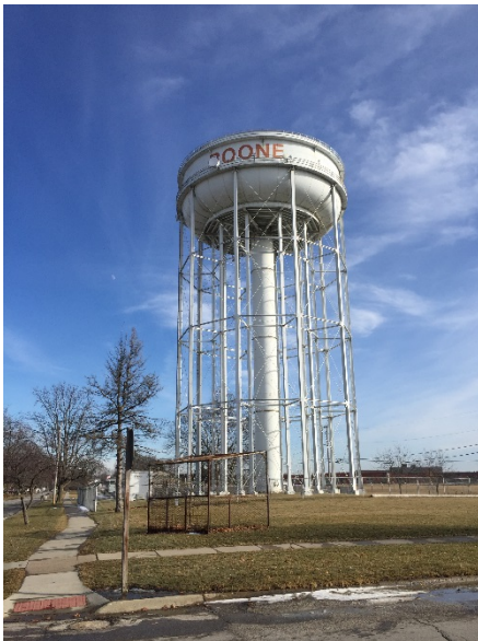
Photo of the tower looking East
