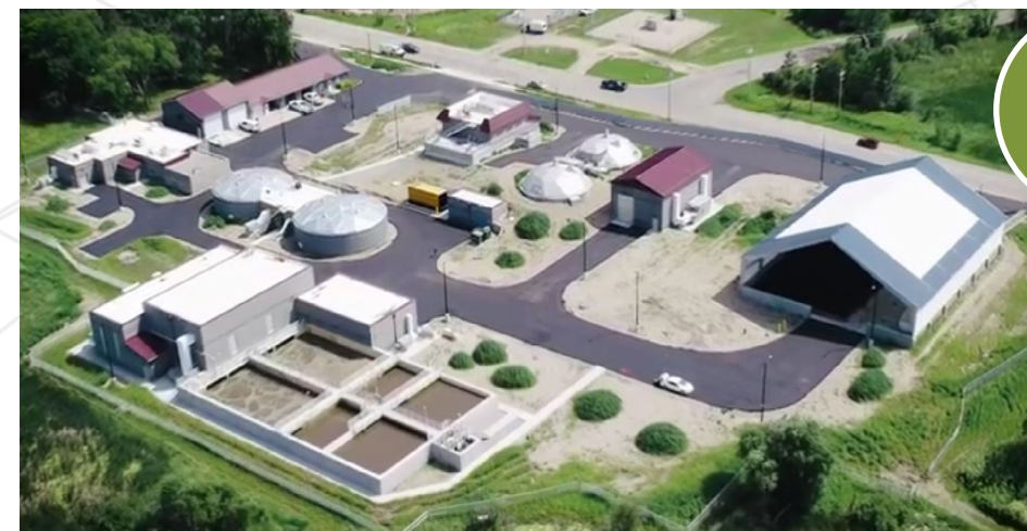
Tackling stringent regulations with one of Minnesota's most innovative facility designs.
