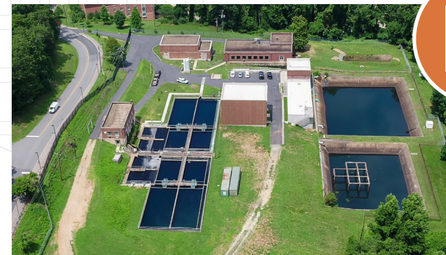
Rehabilitation and expansion of South and Observatory WTPs (Rivanna Water & Sewer Authority)
