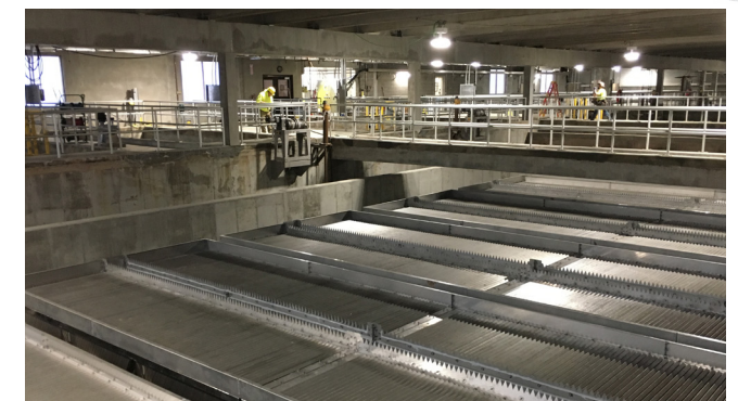
Retrofit of the plant sedimentation basins with high-rate lamella plate settlers
